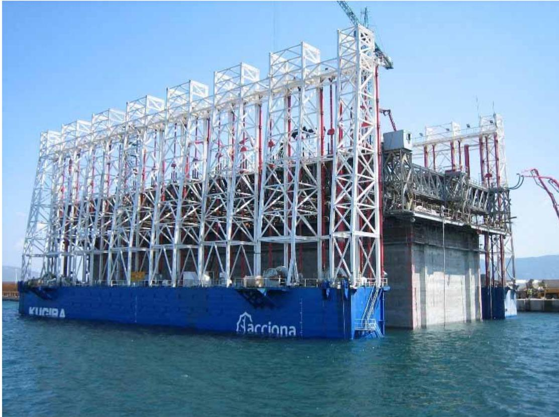
**A system for constructing/placing caisson structures**
